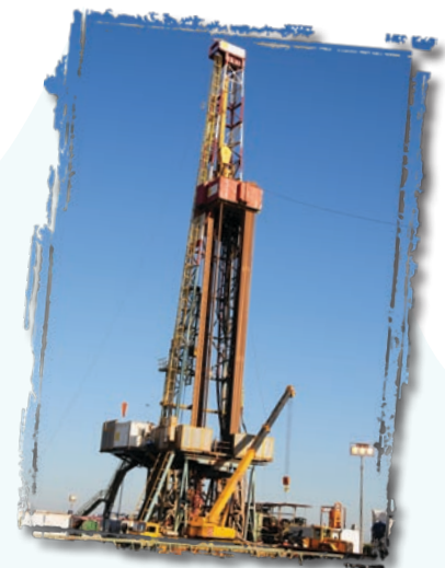
A drilling rig.
