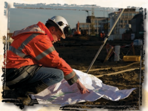
Checking over a construction site.
