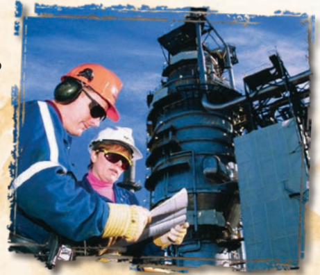
Vacuum distillation unit. Courtesy of Syncrude Canada Ltd.
