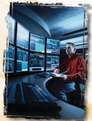
Pipeline Control Centre. Courtesy of Enbridge Pipelines.
